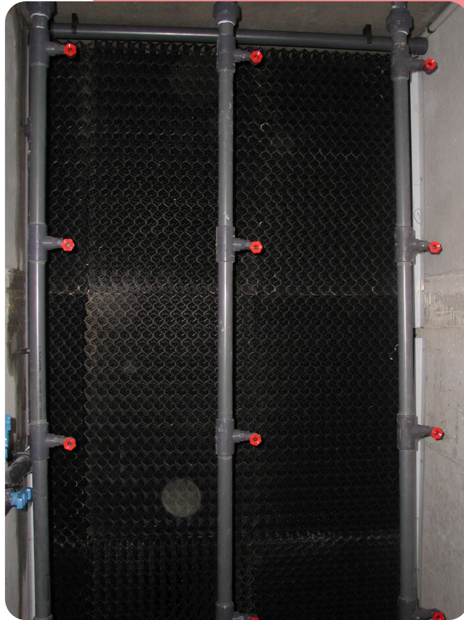
The black mesh at the bottom, and in front are the hollow-cone nozzles.
